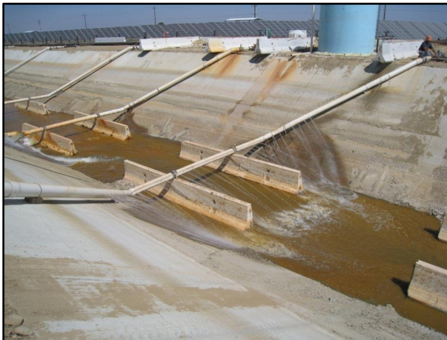
Figure 14-40. Construction of Semitropic Water District Raw Water Processing Facility
