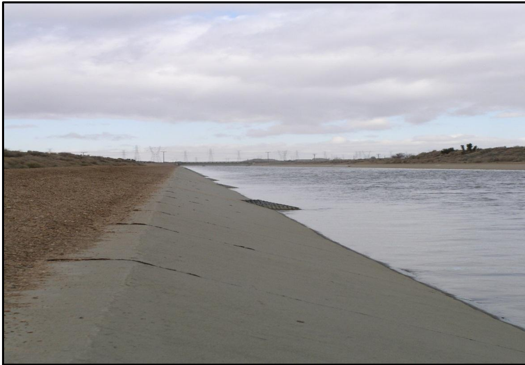
Figure 14-47. Drop Inlets Along the California Aqueduct in Hesperia
