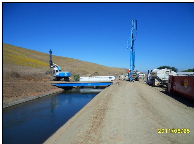
Figure 14-6. New Concrete Farm Bridge with Old Wooden Farm Bridge in Background
